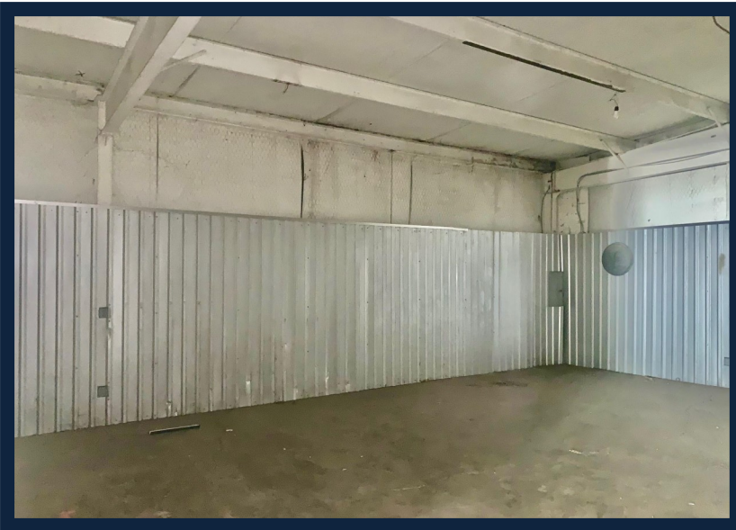
Northeast Corner of Building
