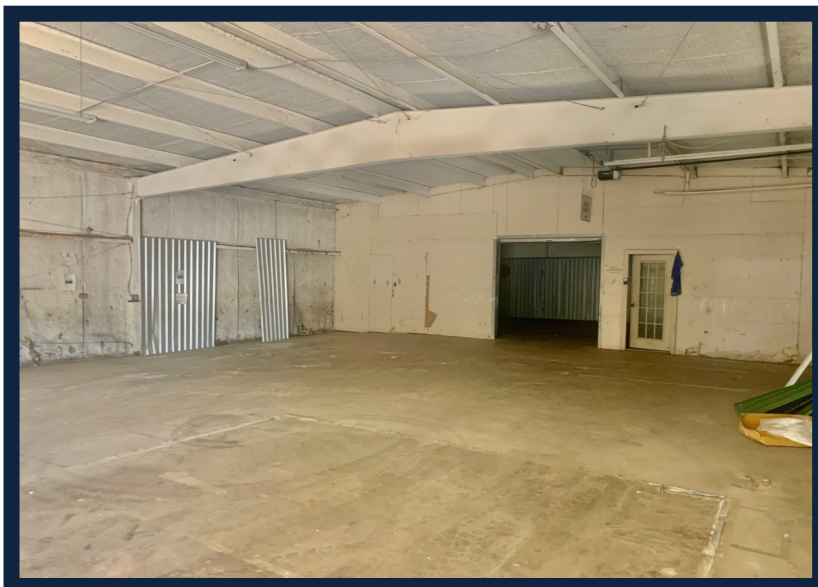
Looking East Through the Warehouse Area
