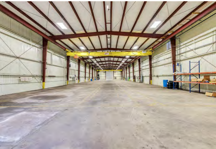
Building 4: (1) 10-Ton + (1) 5-Ton Crane
