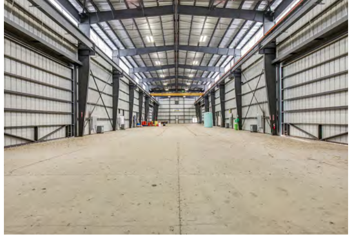
Building 2: 10-Ton Crane
