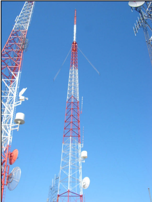
PHOTO OF TOWER
