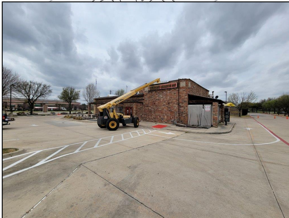
4 : Rear and eastern elevation of building.
