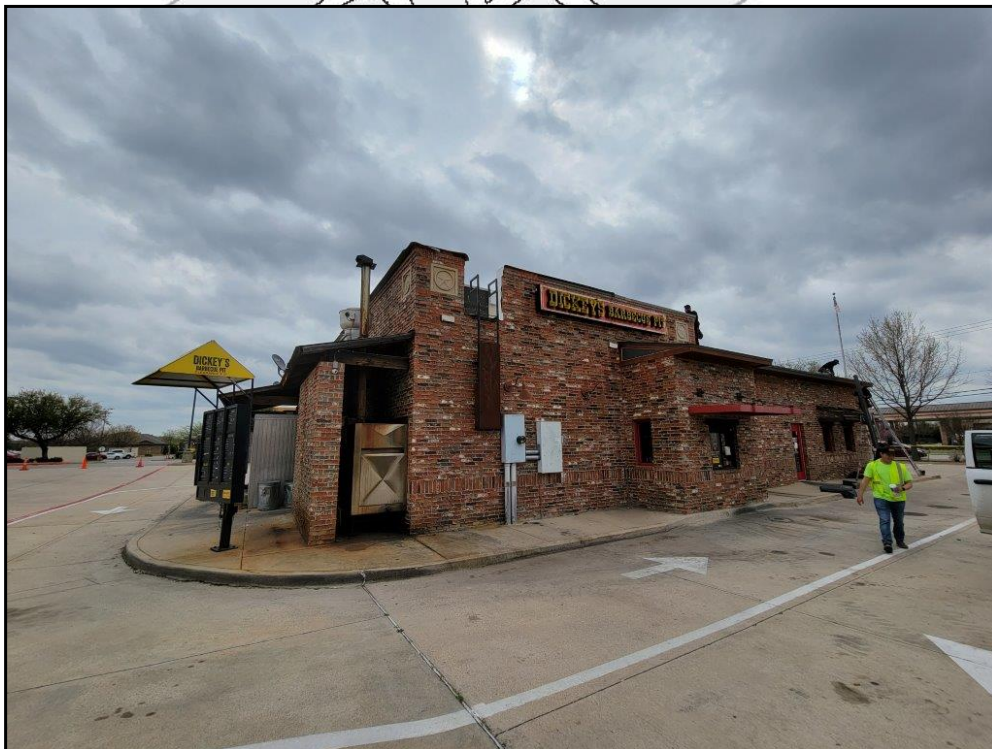
6 : Western elevation of building.
