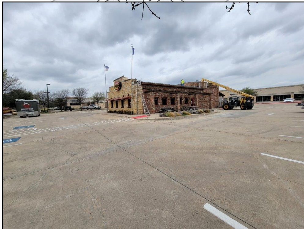
2 : Front and eastern elevation of building.
