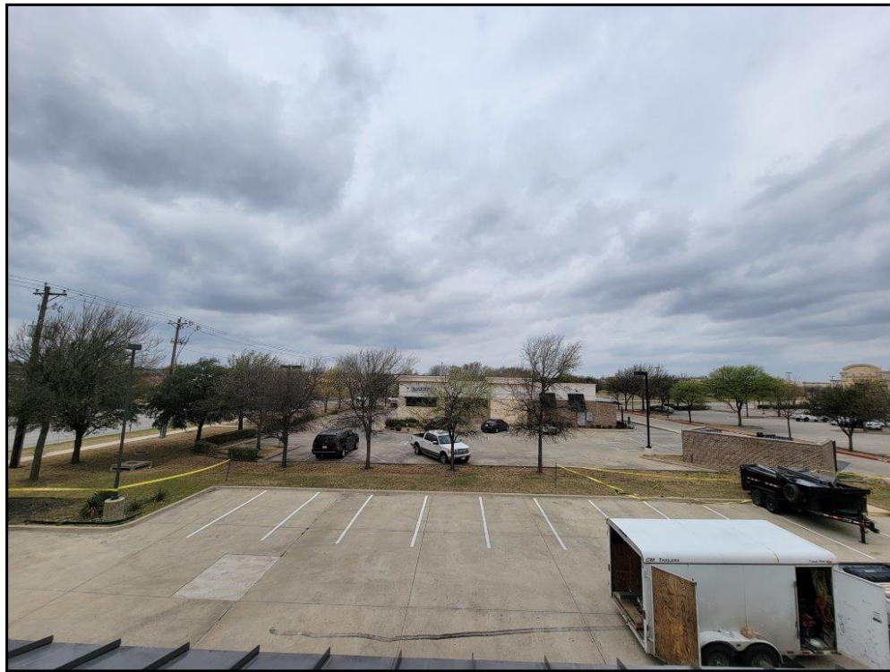
7 : Paving at western side of building.
