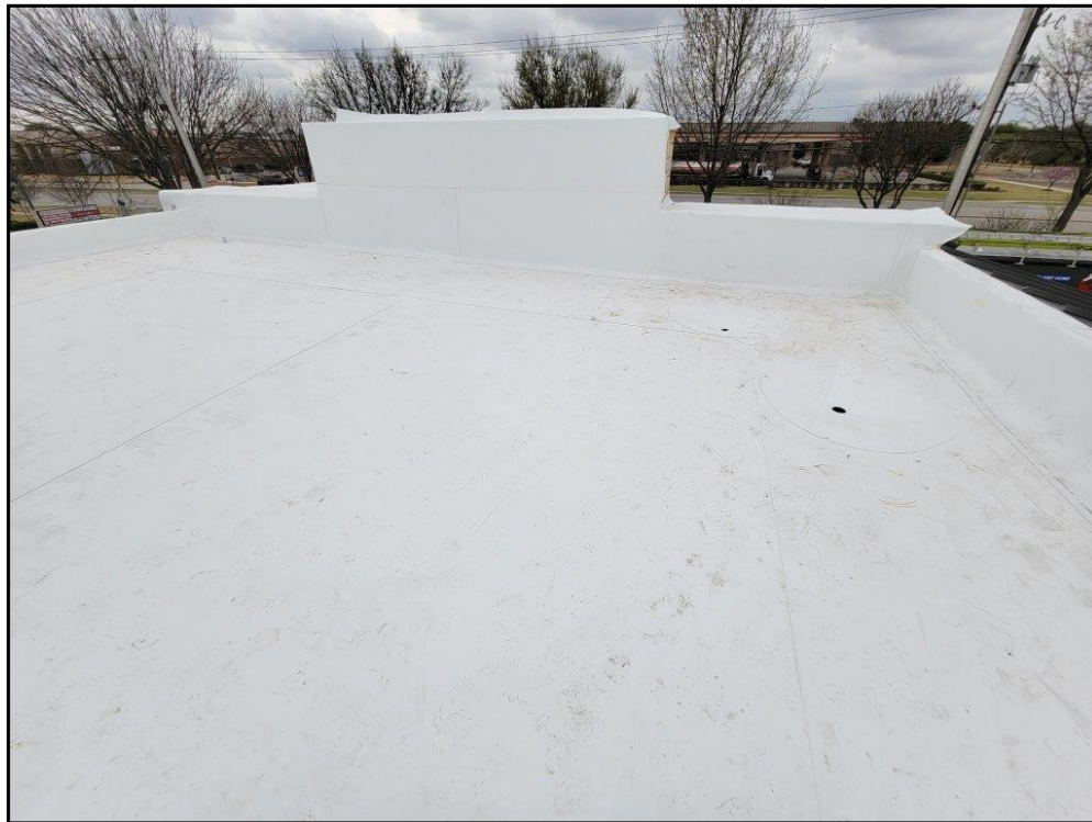
17 : TPO-membrane roofing.
