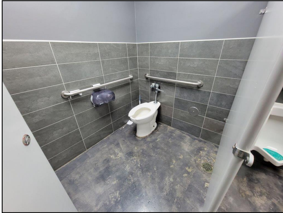
33 : Restroom finishes and fixtures
