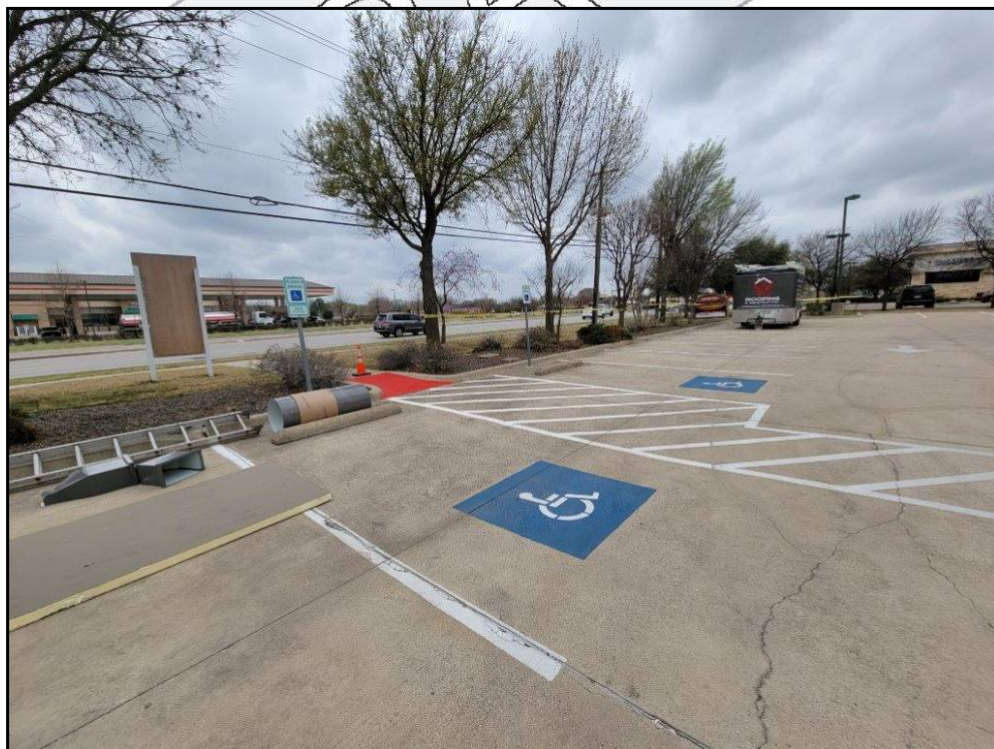
10 : ADA-compliant parking at front of building.
