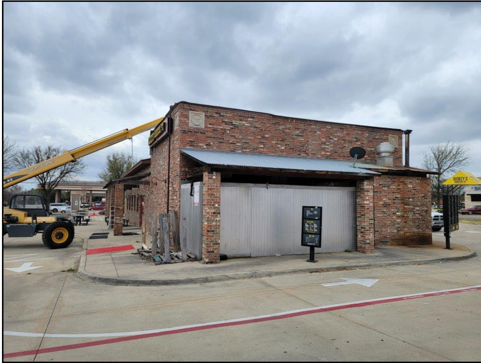
5 : Rear elevation of building.
