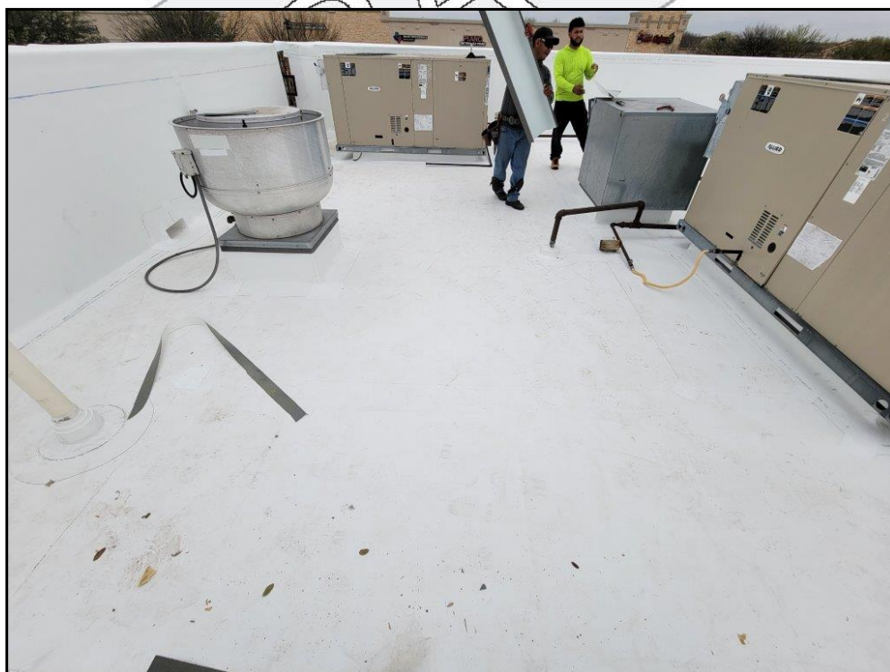
16 : TPO-membrane roofing.
