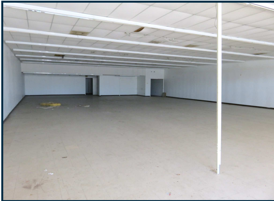
Interior - 5,000 SF (+/-) section
