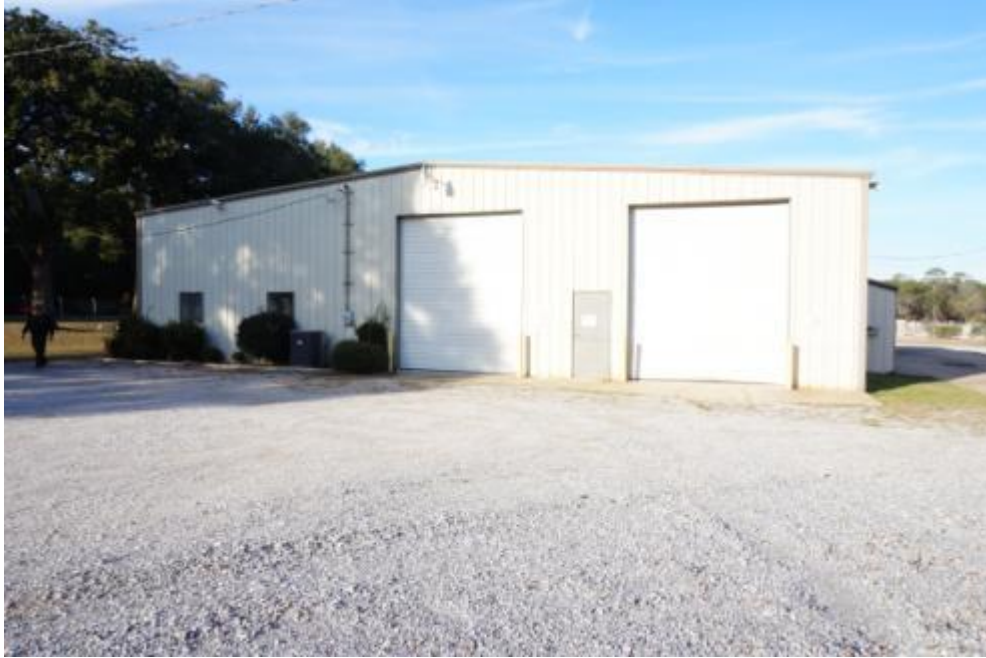
Building 1 (4) Roll Up Doors 12x14' Drive Thru Bays
