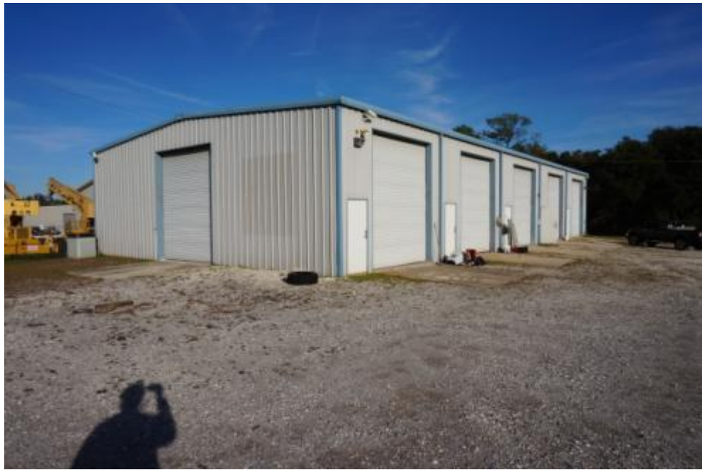
Building 2: has (7) Roll Up Doors 12x14'
