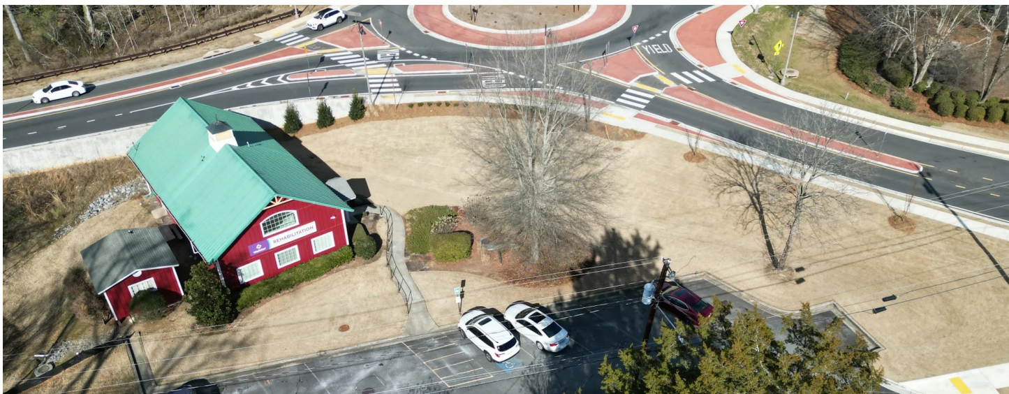
PROMINENT CORNER / ROUNDABOUT EXPOSURE
