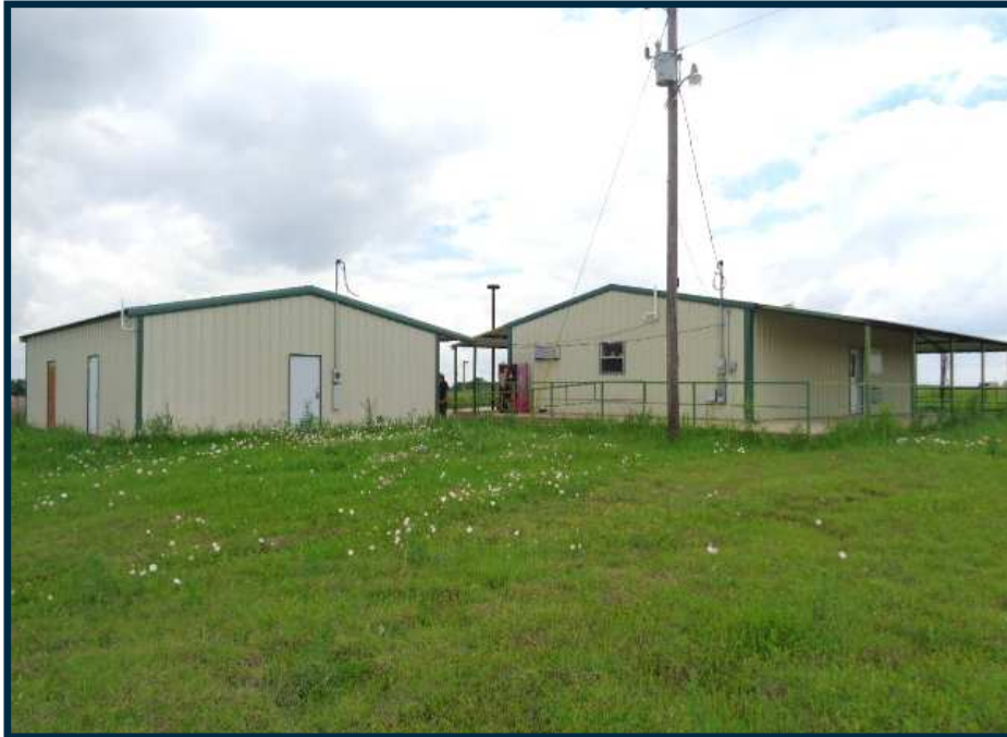
Additional Office/Warehouse Buildings
