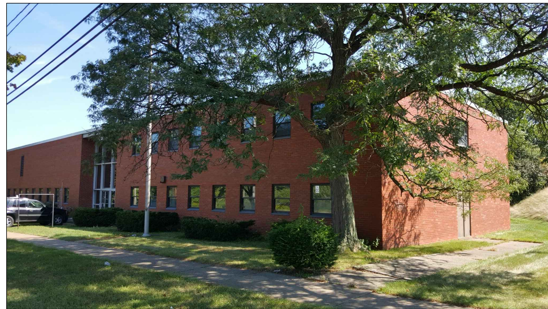
BUILDING FRONT VIEW
