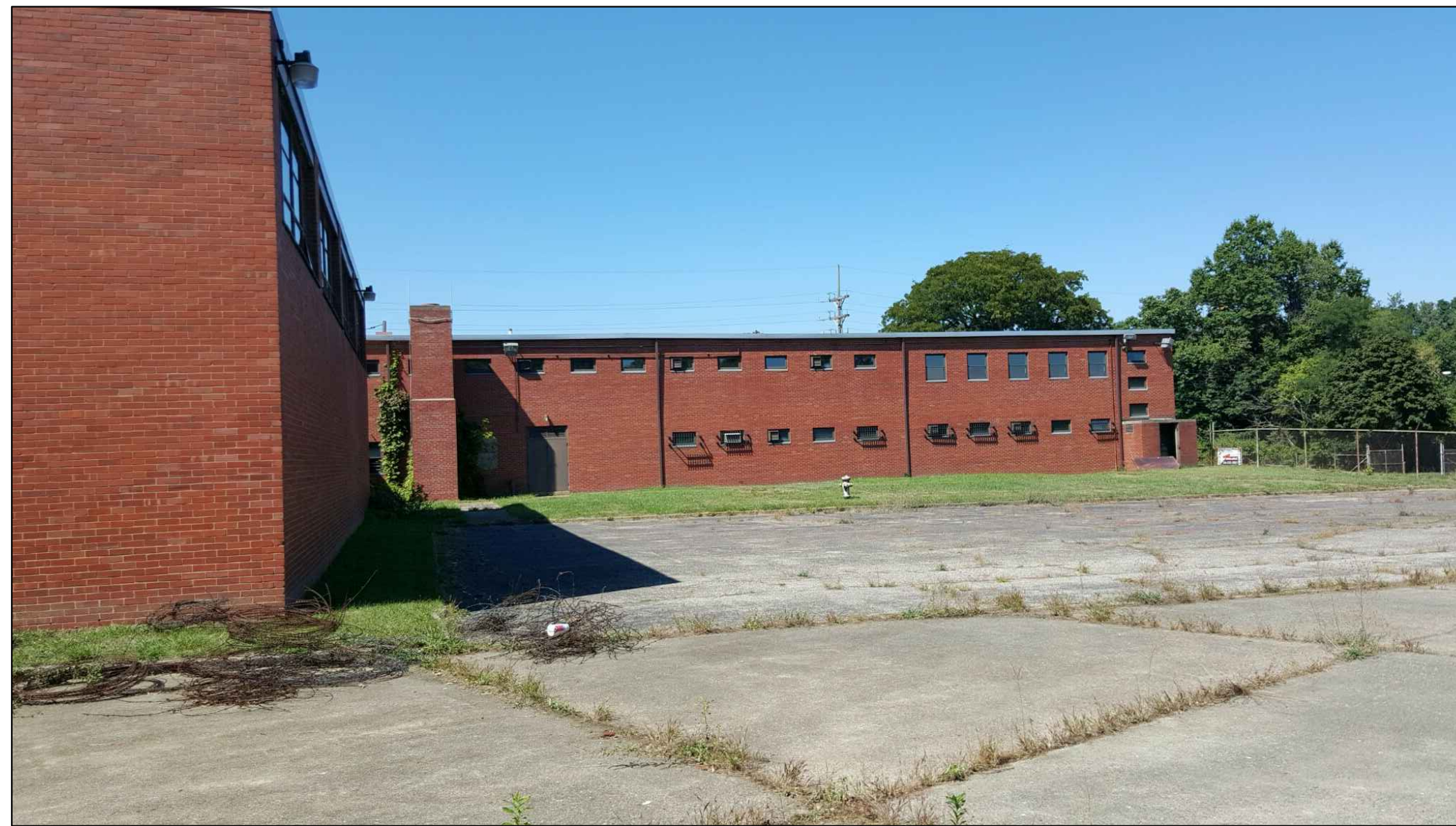
BUILDING REAR VIEW
