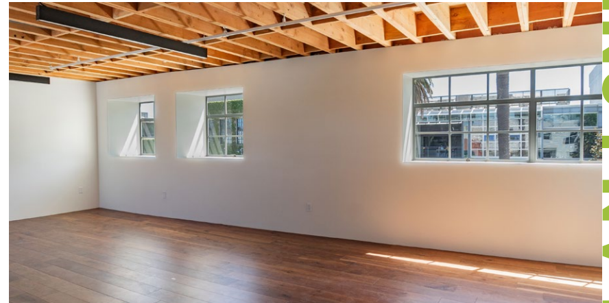
B— MEZZANINE AREA
