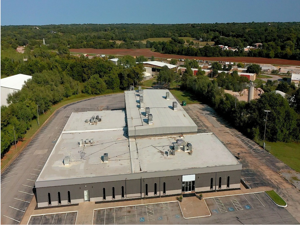
Aerial View of the Main Building
