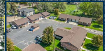
1310 S GARLAND APARTMENTS
