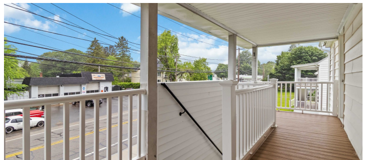
Covered Exterior Access
