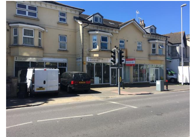
Exterior of building
