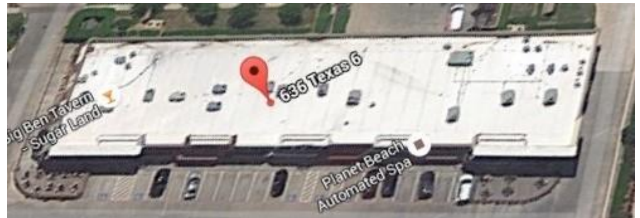
Tilted Aerial View
