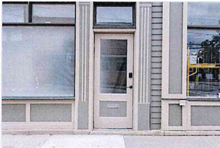
View of exterior entry
