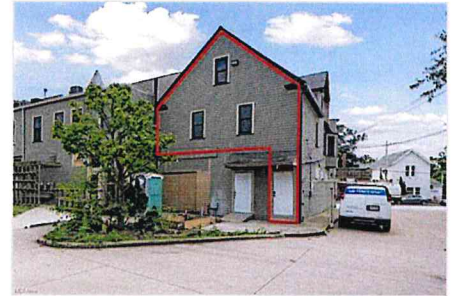
View of front of home
