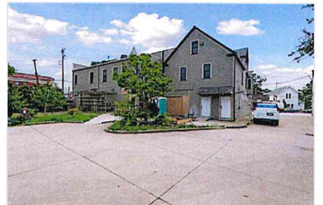
View of front of home
