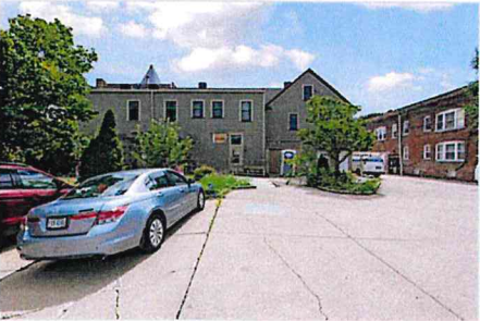
View of road
