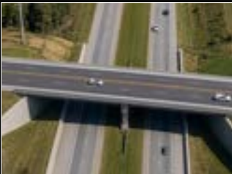
I-65 BRIDGE New Bridge — Master Connector
