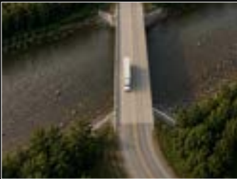
RUTHERFORD CREEK New Bridge — Site Connector
