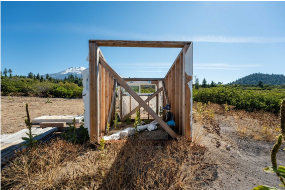
Well head and partially framed enclosure, north end of the parcel
