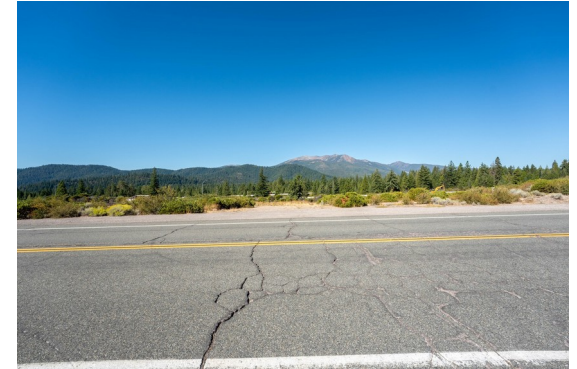
Spring Hill Road frontage at grade
