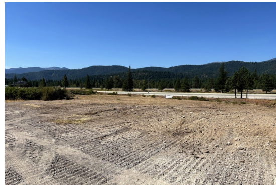
Graded portion of the site, Interstate 5 beyond
