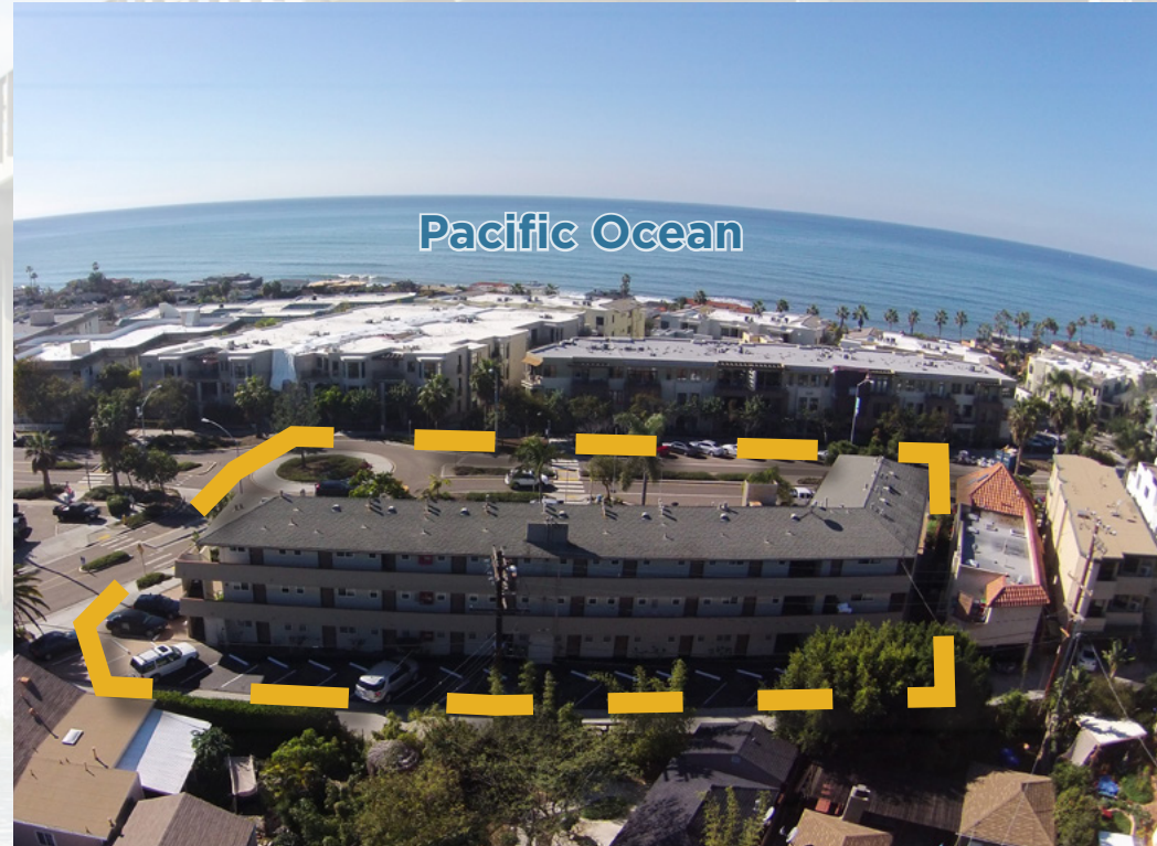
WEST FACING VIEW
