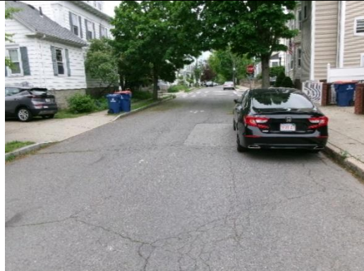
View South on Tremont Street
