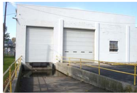
East Receiving Area
