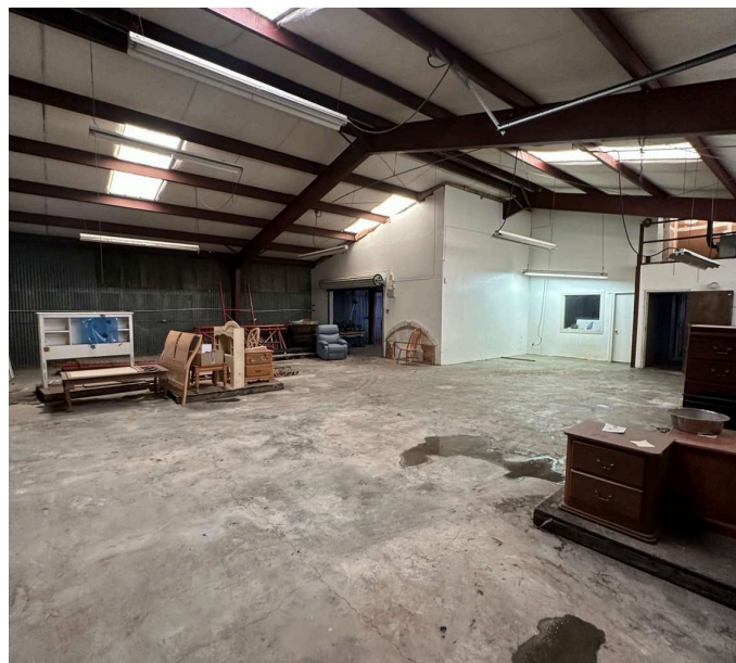
MAIN WAREHOUSE — SKYLIT OPEN AREA
