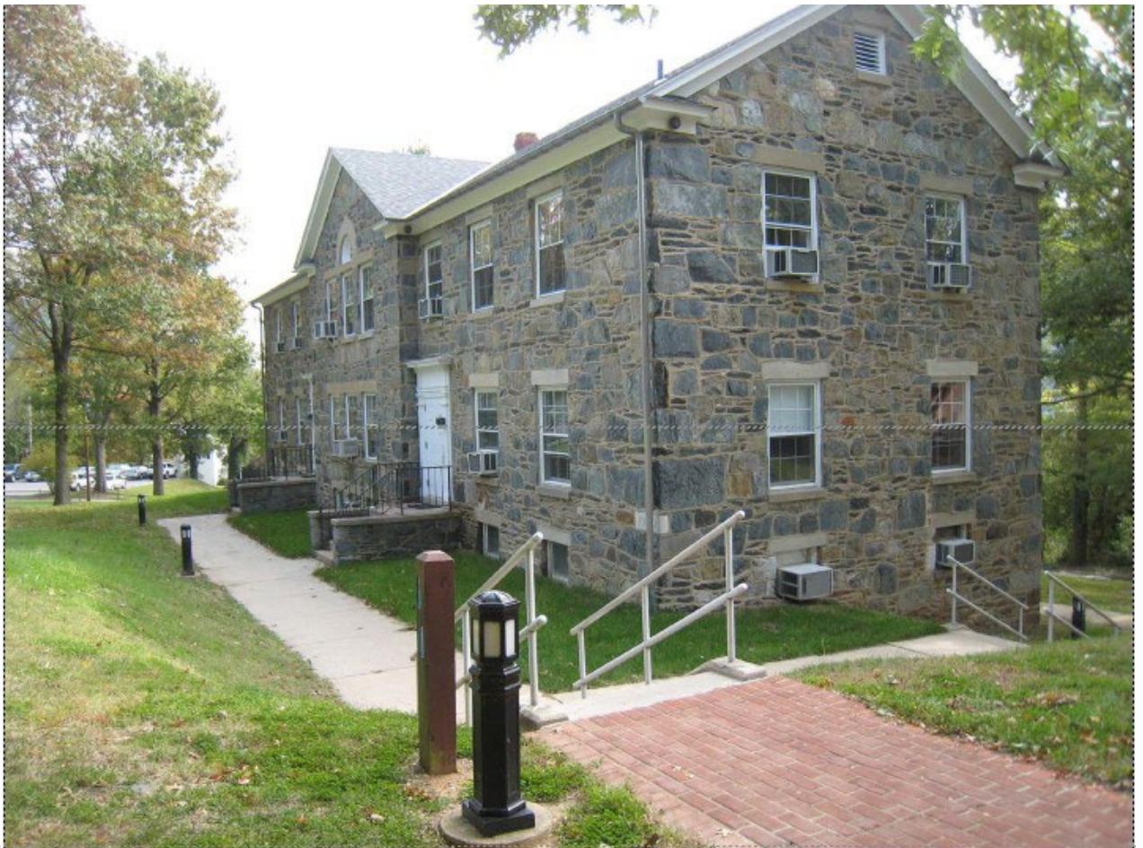
Cook Hall Northwest View (Source: NPS file photo)
