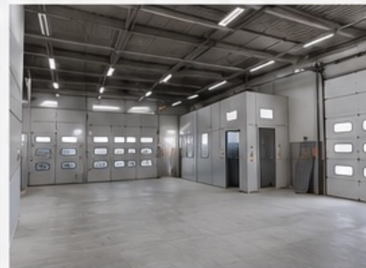
EXPANSIVE PAINT BOOTHS
