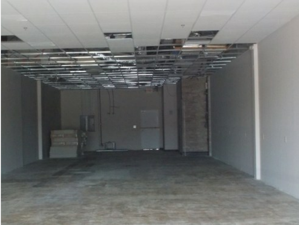
Interior Photo - white box
