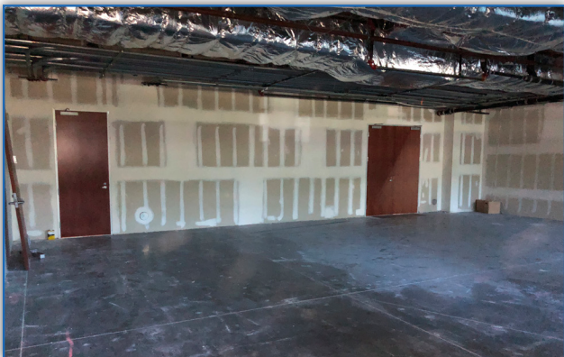
Clean Shell Condition
