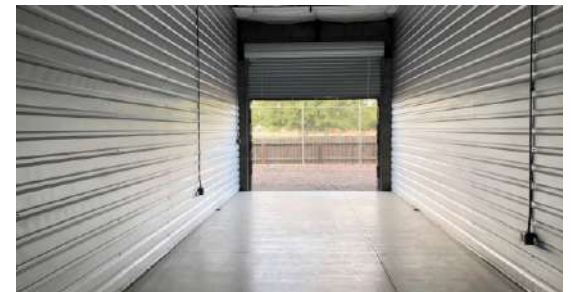
STANDING AT BACK WALL LOOKING OUT
