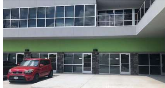
STORE FRONT/PARKING VIEW
