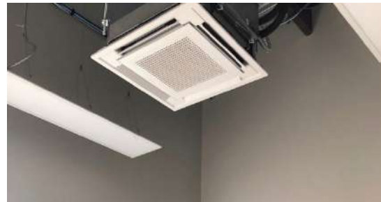
CEILING VIEW OF OFFICE A/C Unit and Light. Height 8.5'
