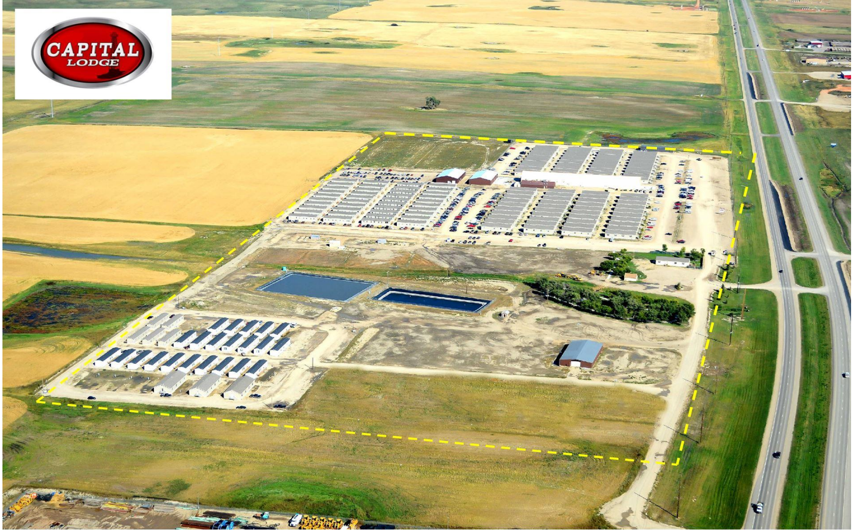
Aerial view of Capital Lodge from the west looking east.
