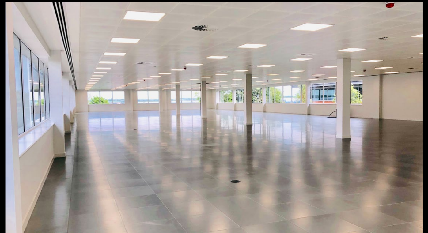
Completed 1st floor refurbishment
