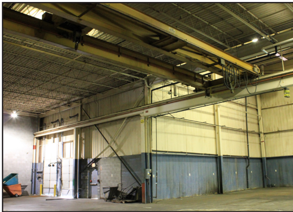
10-Ton Crane to Internal Rail
