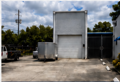
GARAGE & FENCED YARD
