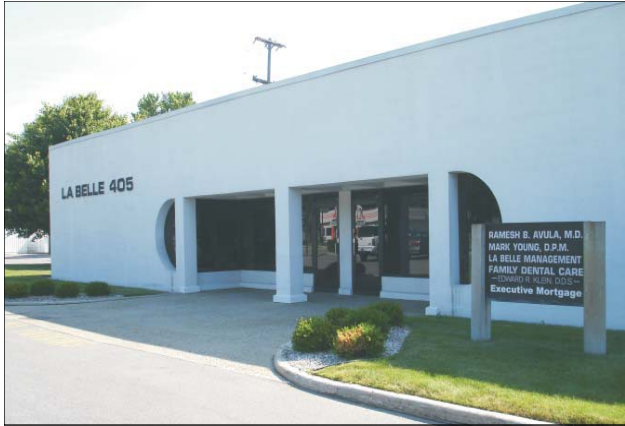
The LaBelle 405 Office Building
