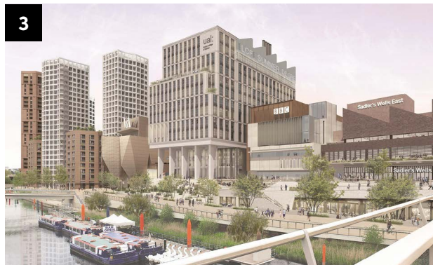
3 East Bank, QE Olympic Park Balfour Beatty & Places for People Phased Completion: Q4 2023/2024
