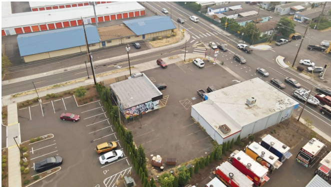
Rear aerial view showing site depth and surrounding uses.
