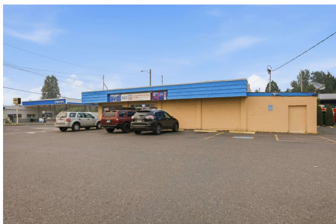
Street-level view of 365 Convenience Store and on-site parking.
