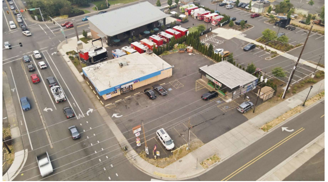
Aerial view emphasizing road access, parking and nearby commercial activity.
