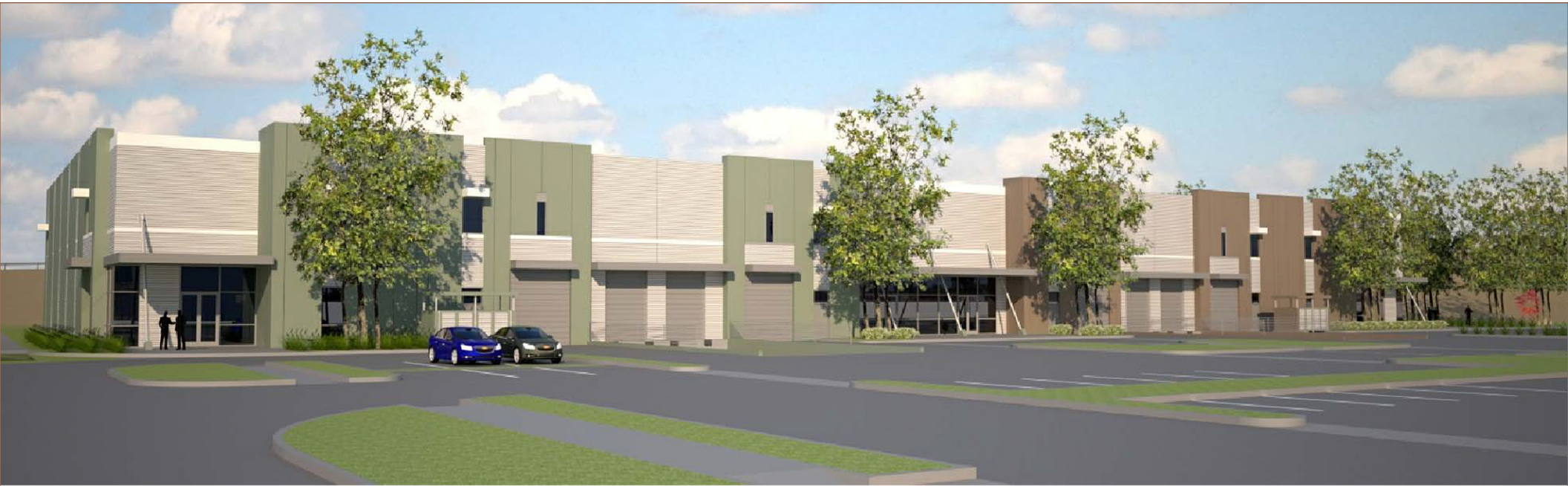
EAST SIDE OF BUILDING
