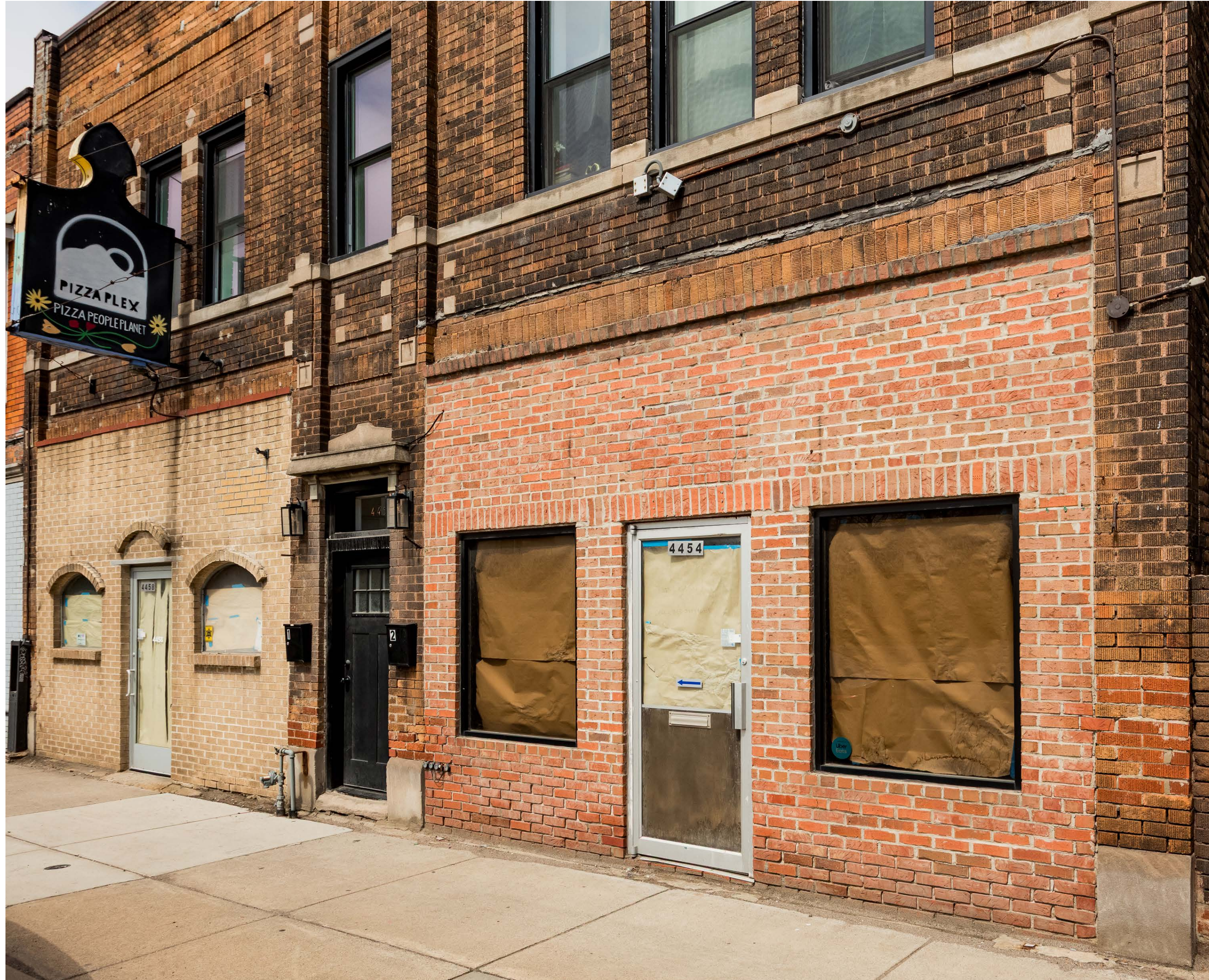
Street-facing storefront with original brick facade and signage potential along West Vernor.
