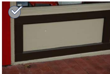
Wood is an appropriate material for replacement of bulkhead if the original is missing.
