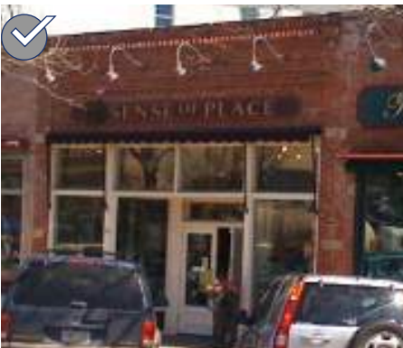
Phase 2: A later rehabilitation effort included removing the stucco, reconstructing the cornice and installing a new storefront system.
