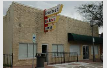
Example of an R3 Structure
