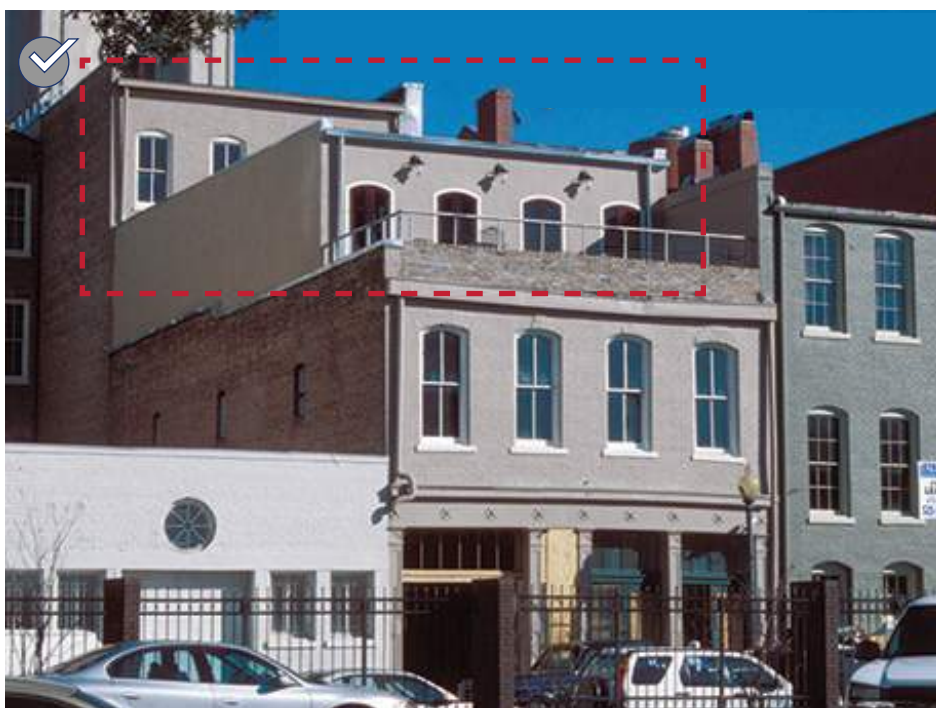
Two-story addition is appropriately setback from the primary character-defining facade.
