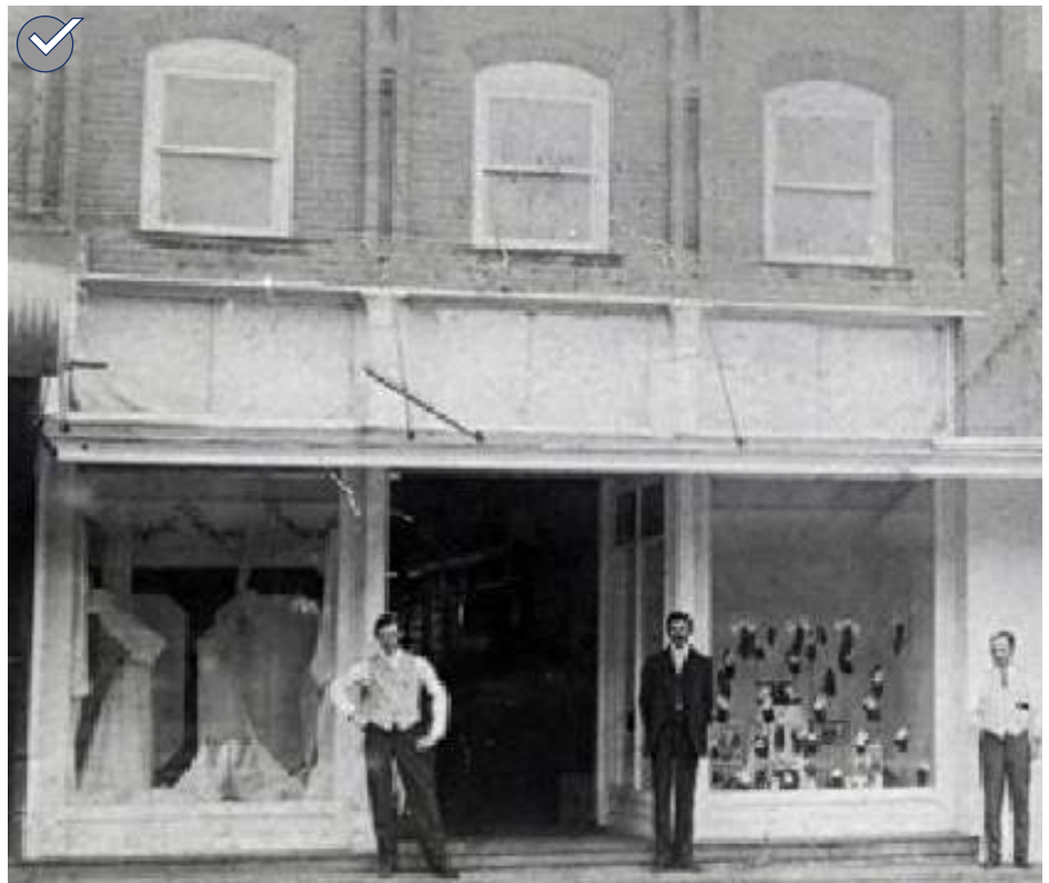
Early storefronts had features typical of traditional commercial buildings: main display windows supported by a paneled wooden bulkhead.
