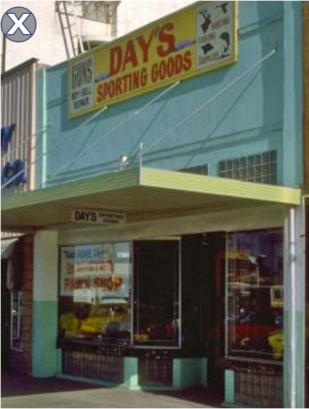
Historic building significantly altered.
