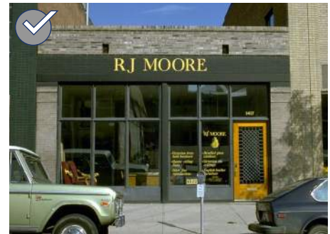
This building illustrates an appropriate contemporary rehabilitation of an altered historic building. The historic structure remains intact and a contemporary storefront has been installed that is in scale with the building.
