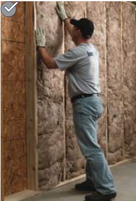
Use noninvasive strategies when applying weatherization improvements. This insulation is being placed on the interior wall.
