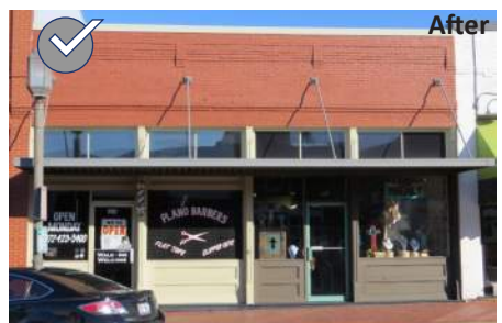
A contemporary storefront should convey the traditional components, such as bulkheads, display windows and transoms, in new ways.
