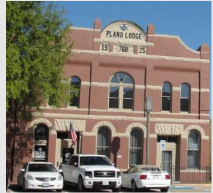
Example of an R1 Structure
