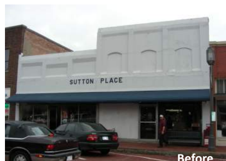
Reconstruction of a key character defining feature, such as this cornice, is a desirable treatment if historic photographic records are available.
