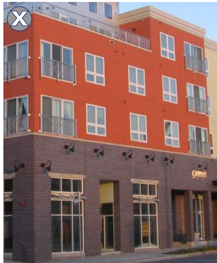
The use of balconettes are inappropriate.
