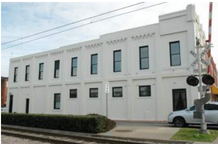
Highly visible secondary wall.
