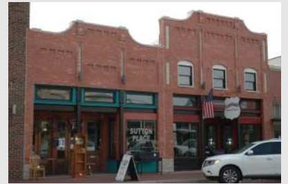
Example of an R2 Structure
