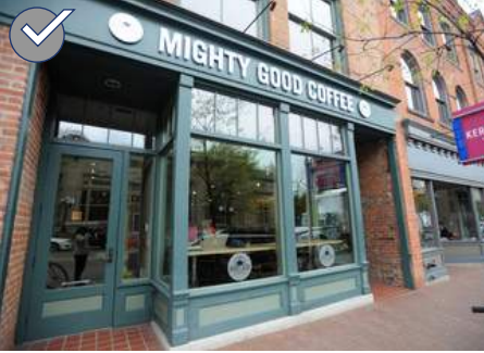
Recessed entries prevent hot and cold air from rushing inside a building when door is opened.
