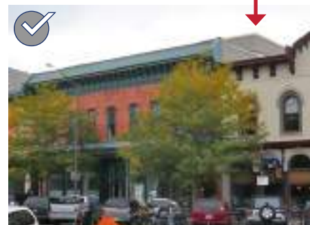
Set a roof addition back from the primary, character-defining facade to preserve the perception of the historic scale of the building.
