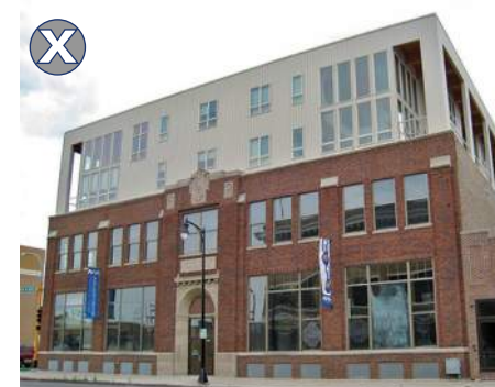
The above and below two-story roof additions overwhelm the existing historic buildings due to its disproportion in mass and scale.
