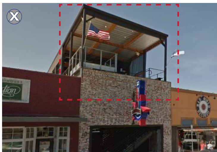
This rooftop addition is set too close to the edge of the historic building wall and impedes one's ability to interpret the historic scale and character of the original structure.
