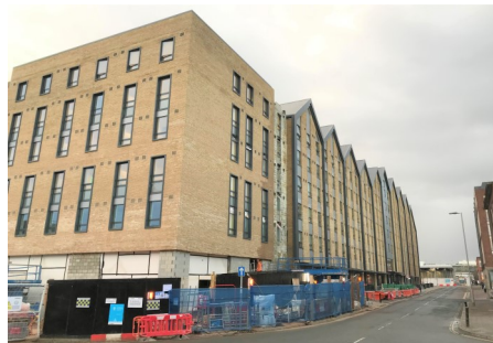
Phase 2 - Summerland Street Under Construction (8/12/2020)
