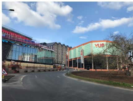
View to The Depot, Vue Cinema & Leisure Centre construction site (12/2/21)
