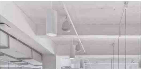
Ceiling Finish - Partially Exposed Concrete Painted White
