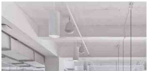
Ceiling Finish - Exposed Concrete Painted White
