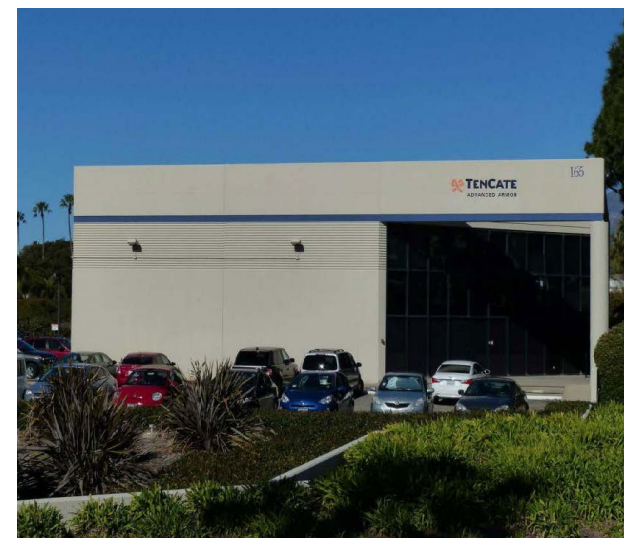
02 – 165 Castilian Drive, building frontage and signage
