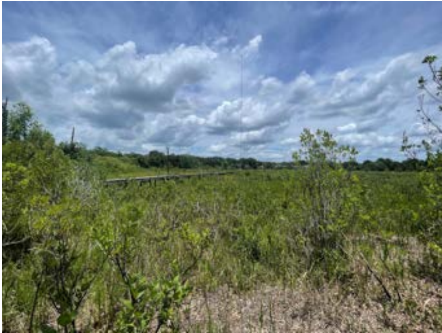
Typical Site View: Access and Inactive Radio Tower in Wetlands,
