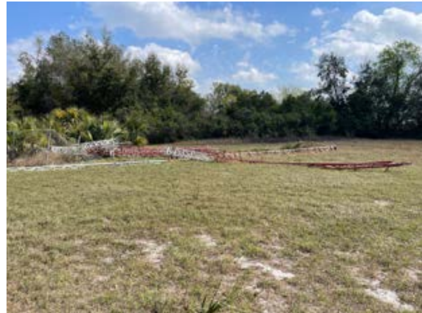
Typical Site View: Debris On-Site
