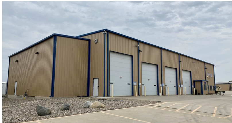
Building 1 | Shop & Office
