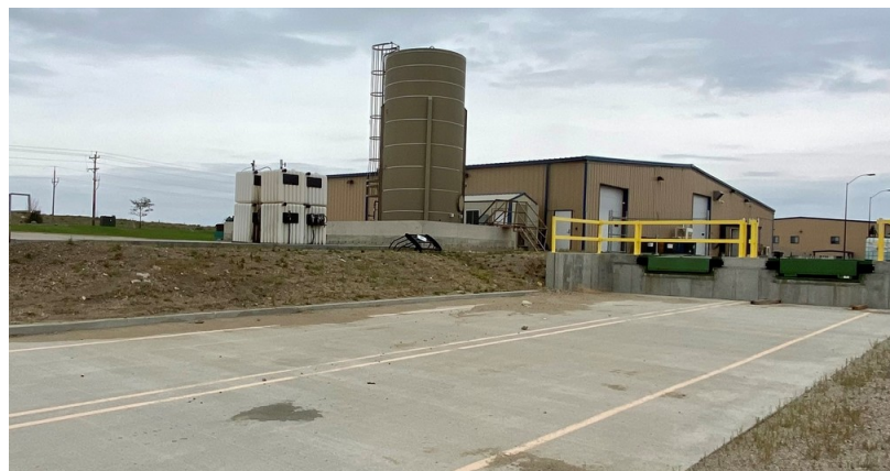
Building 2 | Chemical Warehouse & Lab (Loading Docks)
