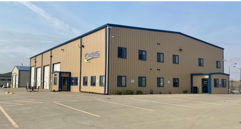
Building 1 | Shop & Office
