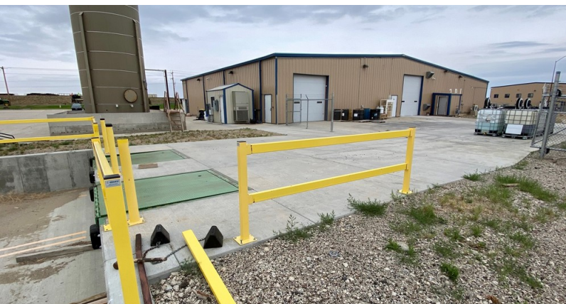
Building 2 | Chemical Warehouse & Lab (Loading Docks)
