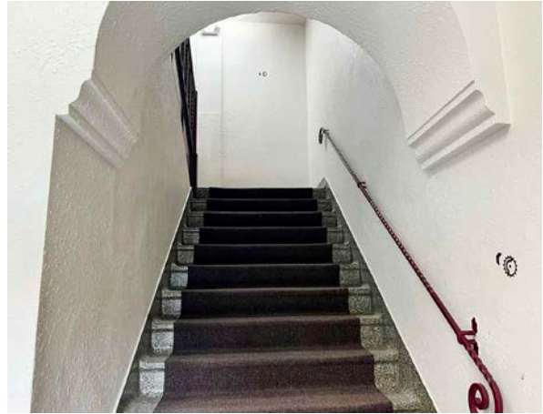
Stairs to Upper Level
