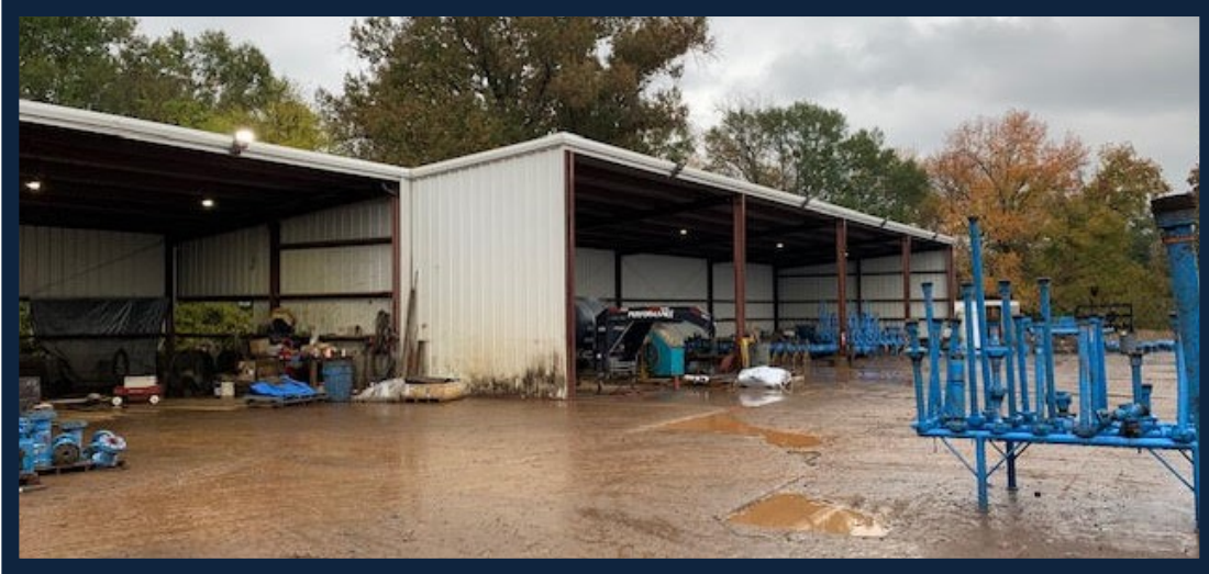
Additional Covered Storage
