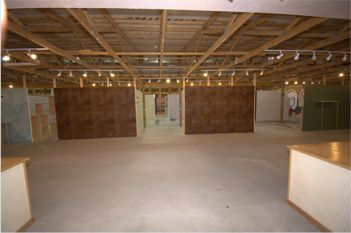
Open-concept interior with exposed wood truss ceiling
