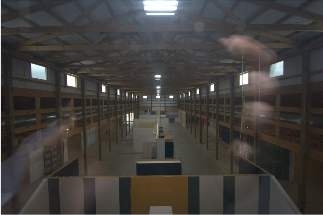
Mezzanine-level view of full building footprint
