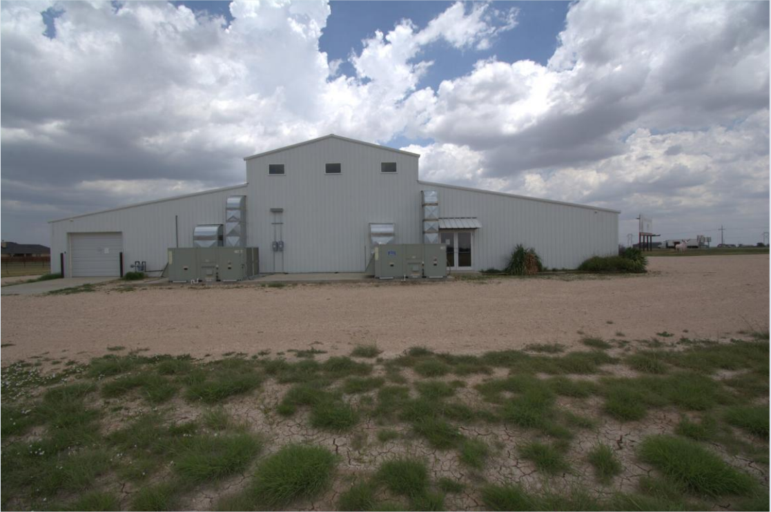
Rear elevation — loading access and mechanical systems
