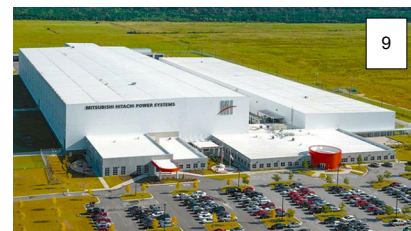
9 MITSUBISHI-HITACHI POWER SYSTEMS
