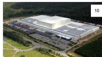
10 IKEA DISTRIBUTION CENTER
