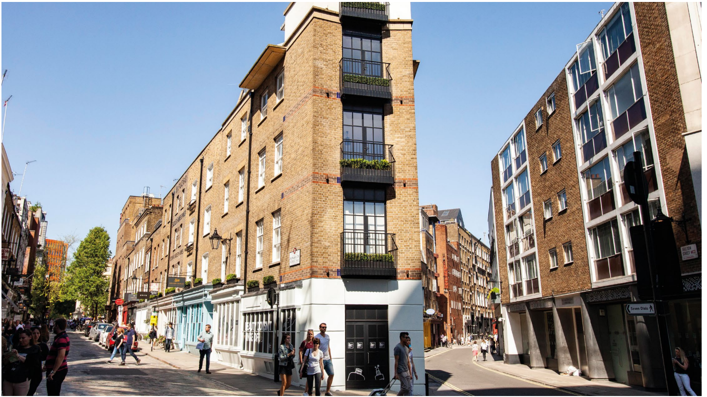
External view looking down Monmouth Street and Shelton Street
