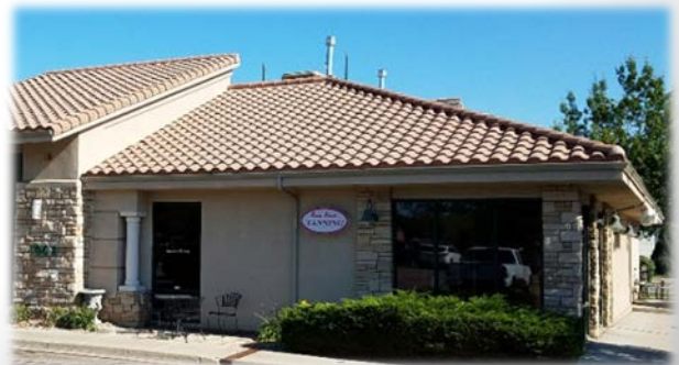
Rental units within walking distance
