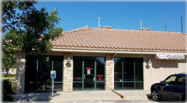
East entry elevation
