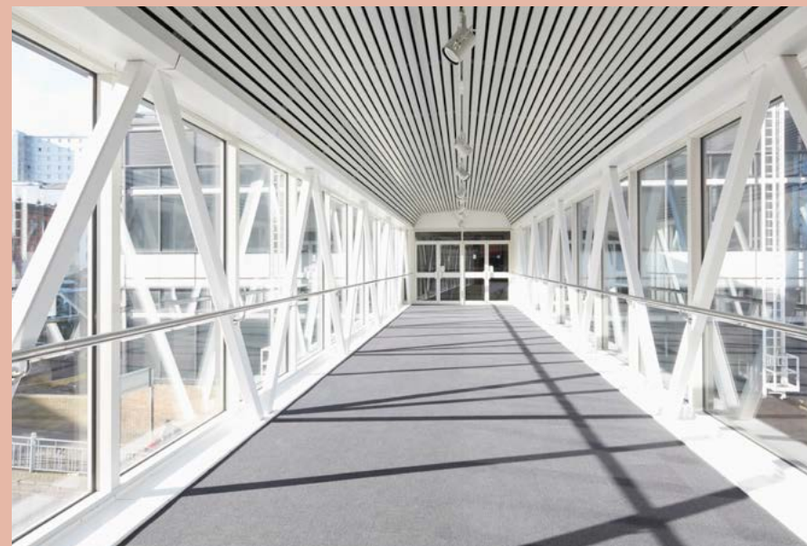
LINK BRIDGE TO READING STATION
