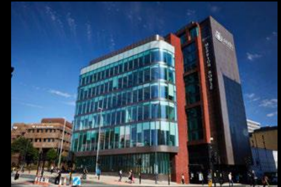
MERRION HOUSE, LEEDS
